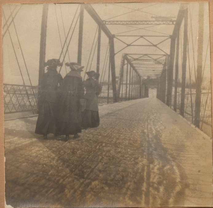
The Windsor Bridge
