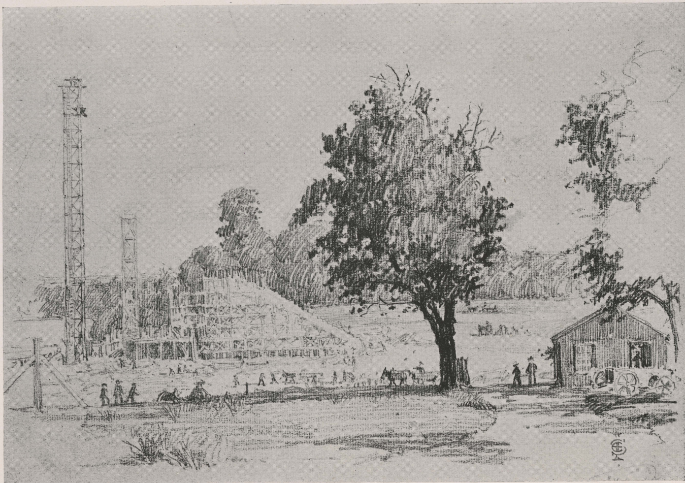
STADIUM IN CONSTRUCTION
