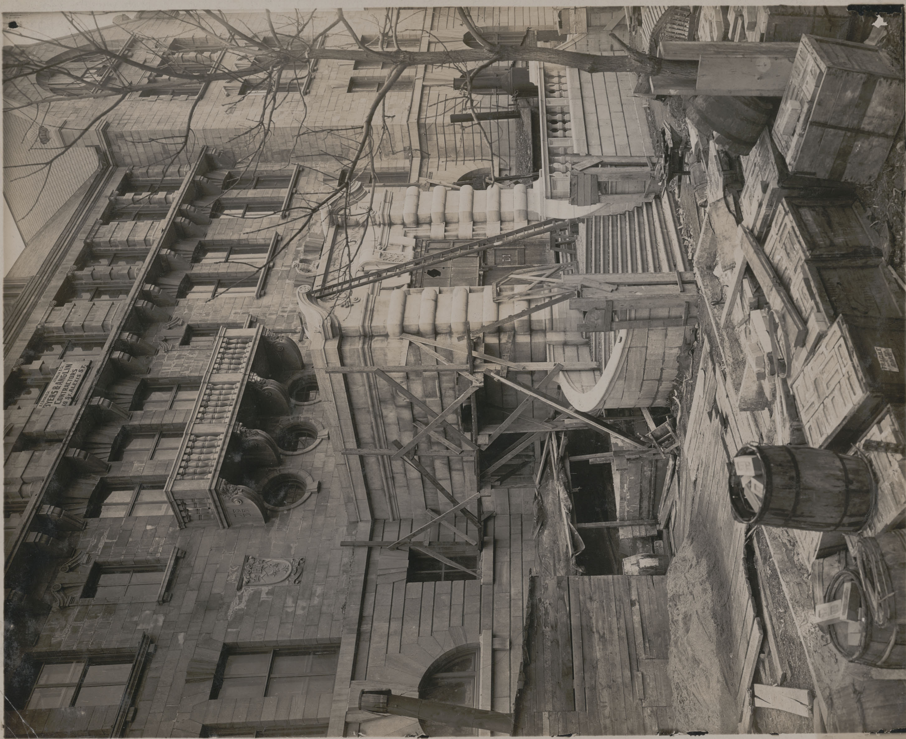
Side View Exterior. McDonald Eng. Bldg.
