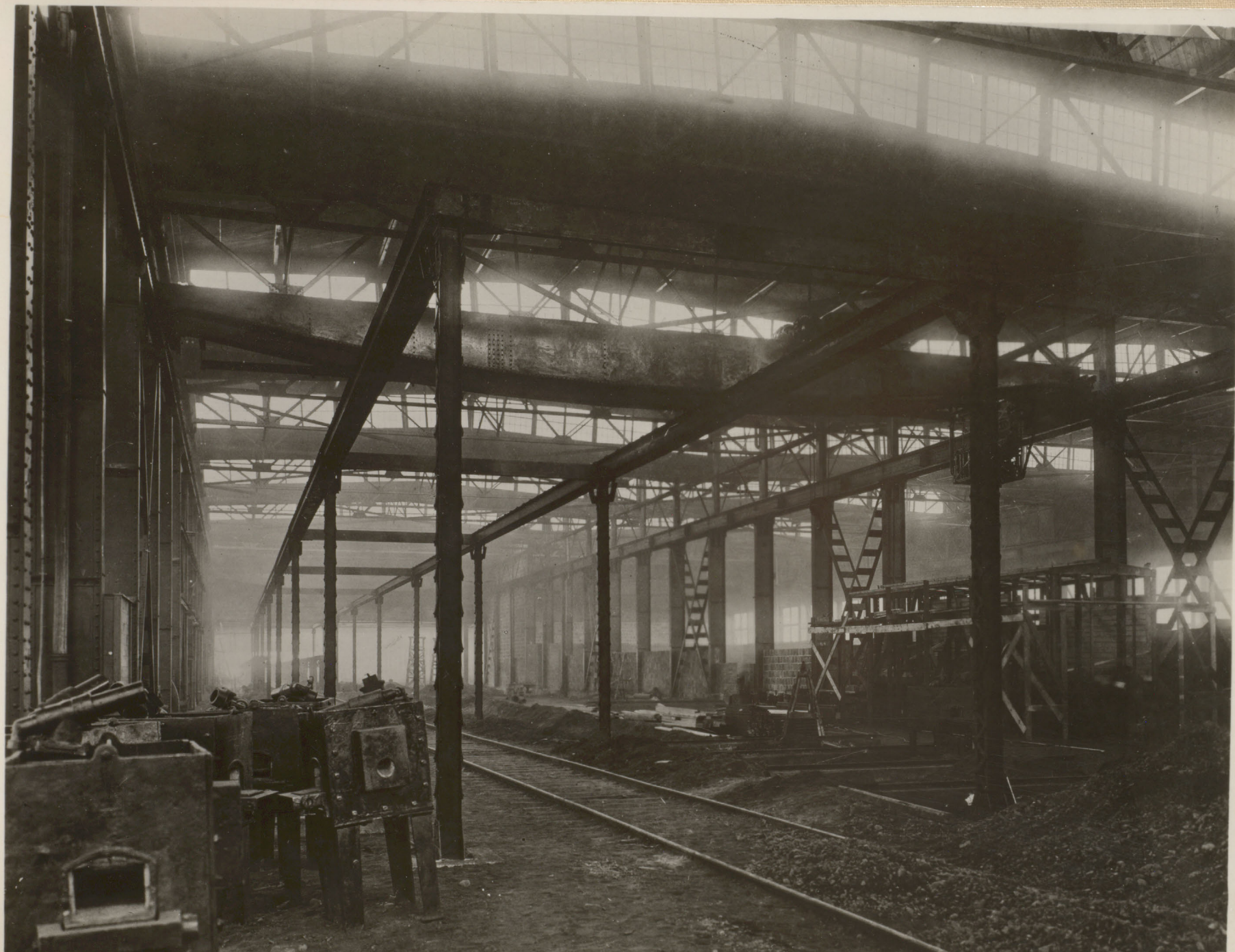
C. C. & F. CO., LTD. FORT WILLIAM PLANT. ERECTING TRACK, AISLE 'B', LOOKING WEST. OCTOBER, 1917. F.P. 19
